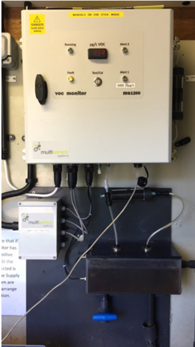
Figure 14. — A picture of the unit installed in the out-building. The unit controls a sluice gate which diverts flow away from the reservoir in the event of contamination
