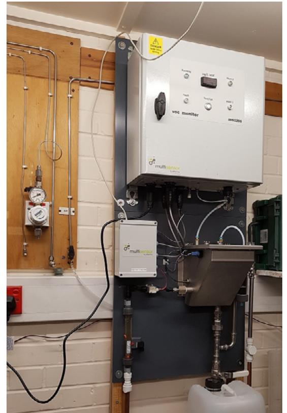
*A picture of the unit installed in the outbuilding. The unit is connected to a PLC that records the data and, in case of an accident, triggers an alarm that switches off the intake pumps.*
