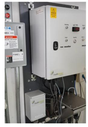
Photo showing the MS1200 installed in the Pump Station. The unit is connected to a SCADA system (Ethernet) using the Profibus Protocol (TCP / IP), which records the data and, in case of an accident, activates the alarms that shut off the suction pumps.
