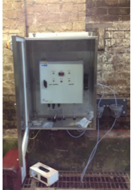
*Unit installed in a wastewater plant in Scotland to detect high levels of VOCs*
