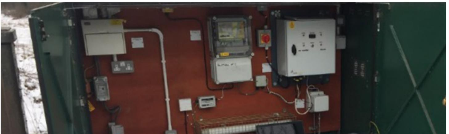
*Unit installed in a cabinet. There are 6 of these cabinets on the industrial estate and include heating system, lighting protection and connection to the telemetry system.*
