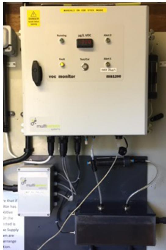
*A picture of the unit installed in the outbuilding. The unit controls a sluice gate which diverts flow away from the reservoir in the event of contamination*
