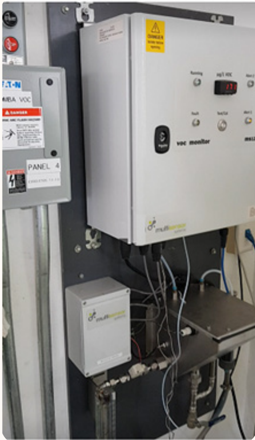
Photo showing the MS1200 installed in the Pump Station. The unit is connected to a SCADA system (Ethernet) using the Profibus Protocol (TCP / IP), which records the data and, in case of an accident, activates the alarms that shut off the suction pumps.
