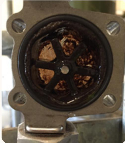
**Before the installation of the MS1200 on-line VOC analyser this is the kind of damage that was often done to the membranes.**
