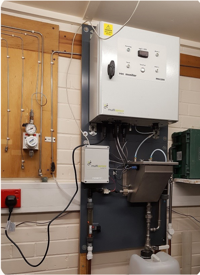
A picture of the unit installed in the out-building. The unit is connected to a PLC that records the data and, in case of an accident, triggers an alarm that switches off the intake pumps.
